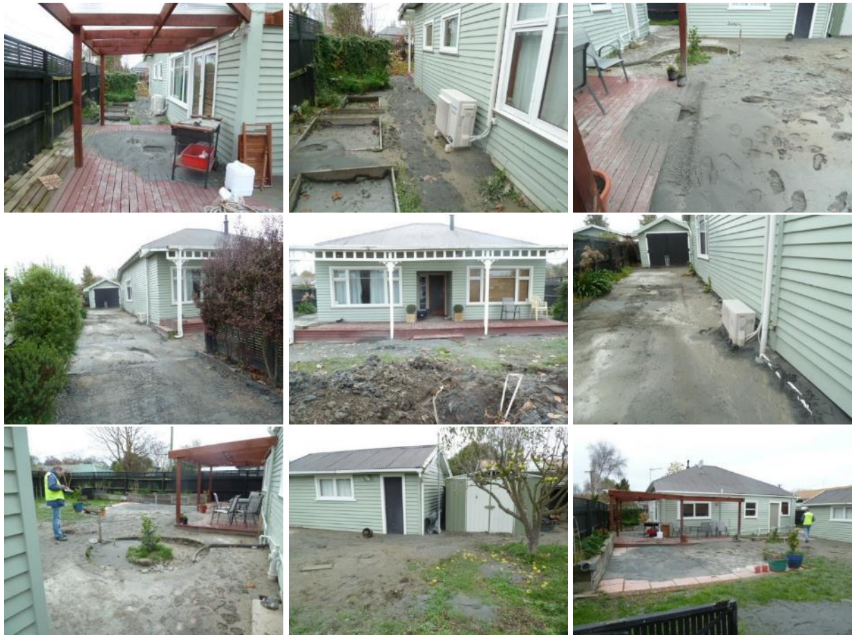
Figure 42: Ground photographs showing ejecta at the property with Patch A (photograph date: 22 June 2011).
